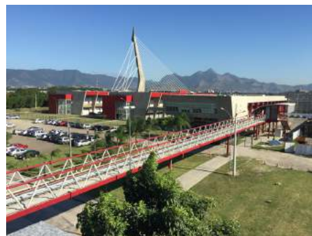
(b) Via elevada
